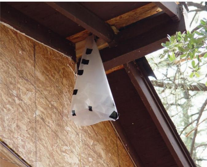
Open-bottom screens and self-made sleeves are effective and affordable tools that prevent re-entry to the roost, while also allowing interior bats to exit.
