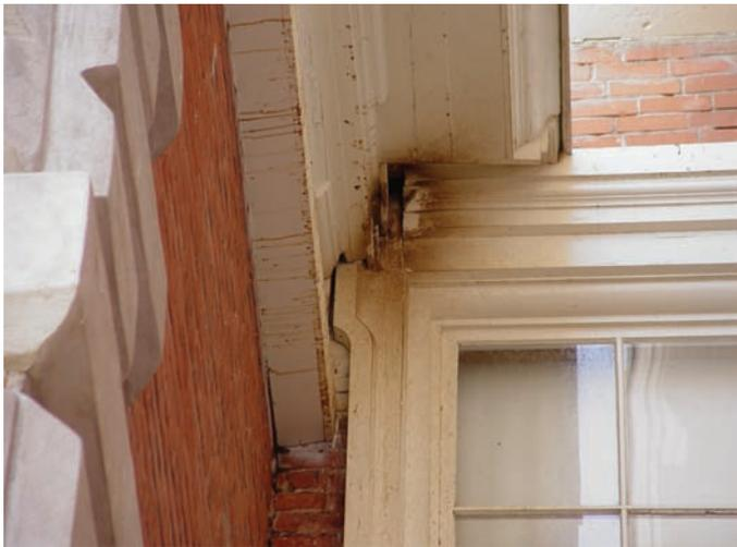
A halo-like rub mark around an entrance hole reveals a bat roost; guano accumulates below a frequented roosting site; a white urine stain in a corner beneath a roost.
